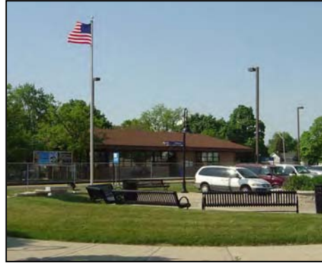
Mokena - Front Street Station
