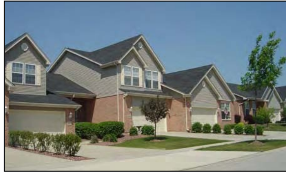
New Residential Housing Construction in Mokena
