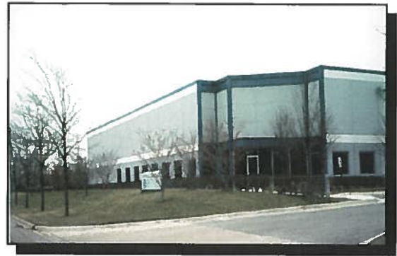
Example in which building design has minimal roof articulation and presence of large blank walls that should be avoided in future designs.
