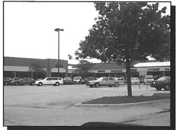
The monotonous image of commercial strip centers, as depicted above, can be improved through the introduction of vertical or horizontal design elements and/or roof articulation.
