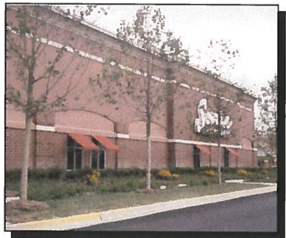
False windows and window awnings are an effective means of minimizing the visual scale of exterior wall surfaces.
