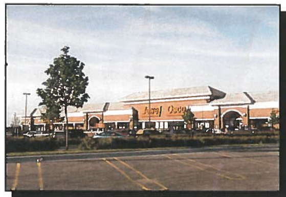
Variations in roof lines help to reduce scale and add visual interest.
